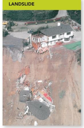
Earthquake shaking can be strong enough to cause soil and rock on a hillside to slide down the slope. A landslide can rip apart homes at the top of the slope and also crush homes at the bottom of the slope.
