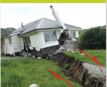
A strong earthquake can cause the two sides of a fault to suddenly slide by one another. Even a relatively minor fault rupture can cause foundation and structural damage requiring expensive repairs.
