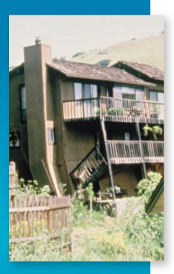
The balcony of this hillside home partially collapsed and the home tilted when the stilt-type support posts and poorly braced walls shifted during an earthquake.
